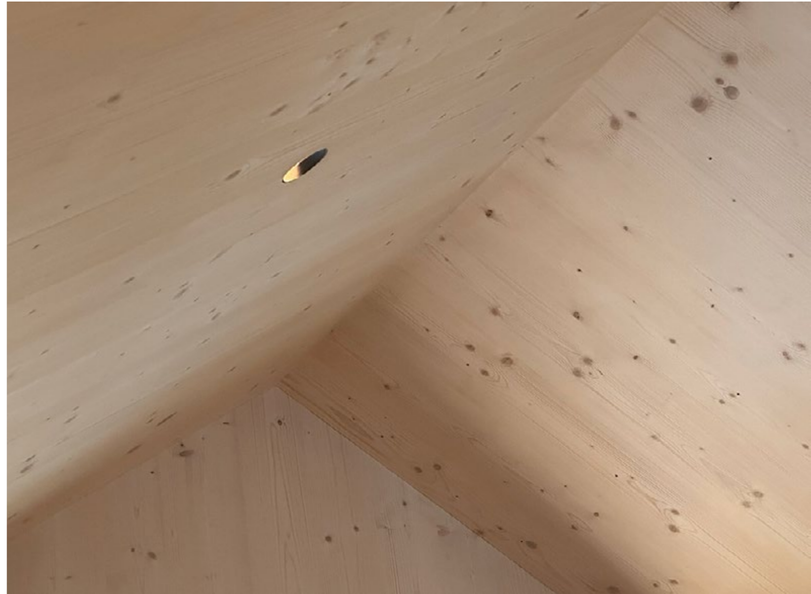
Finished product in the ceiling
