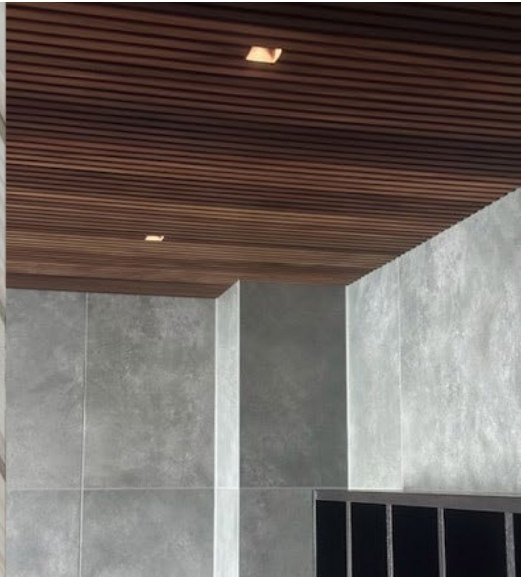
Finished product in the ceiling
