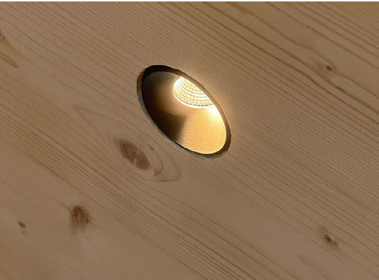
Finished product in the ceiling
